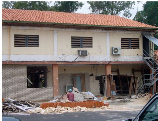
Renovation at SEAM
