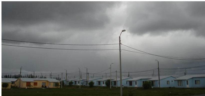
The houses for the workers during the construction period
