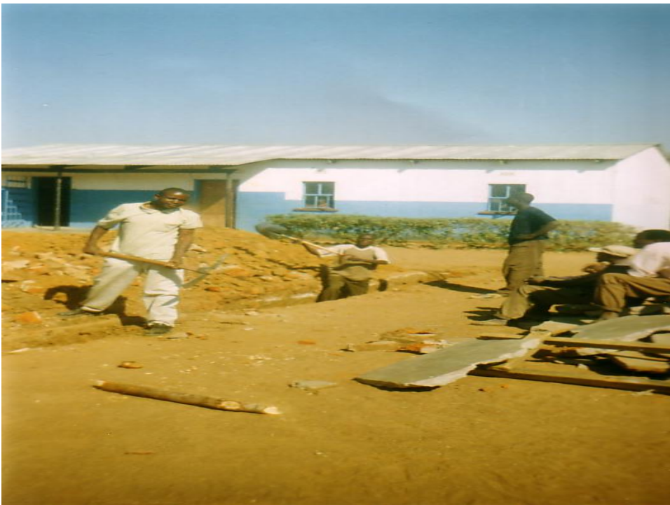
Plate 5: Community initiative project to expand the school
