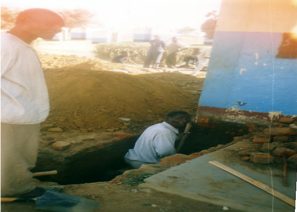
Plate 6: Community members working on expanding the school
