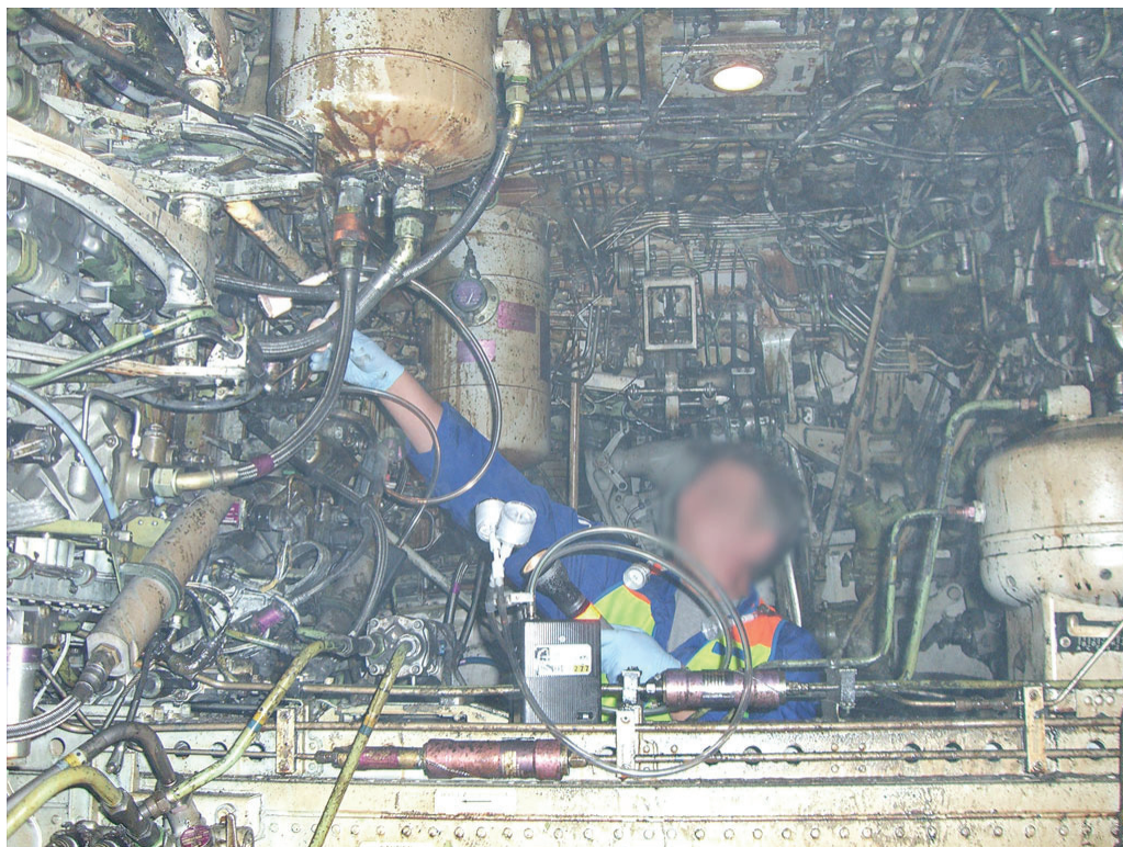
Figure 2-13: Pressure drop of hydraulic system prior to wheel well maintenance.
