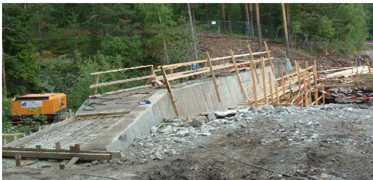
Figure 1.4: Årbogen Dam during the rehabilitation in 2003
