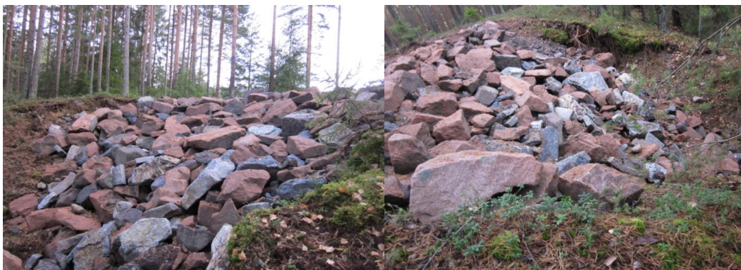
Figure 1.1: Two main slides happened at the Årbogen Dam site.(Captured during the field visit on 28th October 2010)
