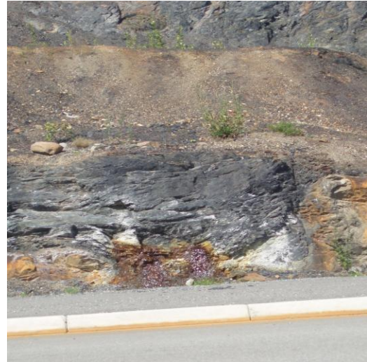
Figure 4-30 water leaking through alum shale
