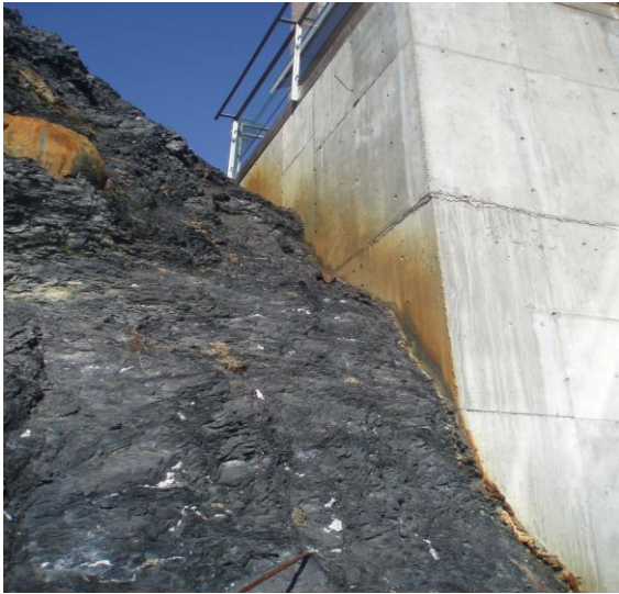
Figure 3-1 A building in contact with the alum shale of the Slemmestad area from which samples were taken
