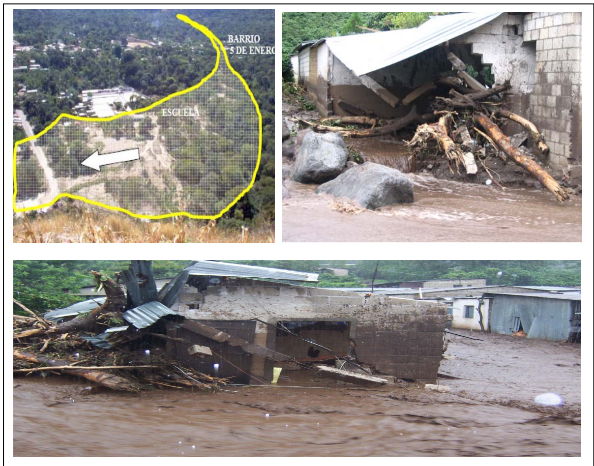
Fig.7.2. Picture of the deposition area (top right). Pictures of the streamflow and the damage it caused in the San Juan La Laguna community.
