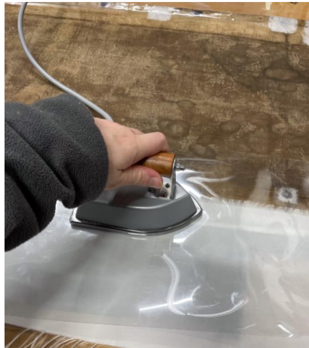
Fig. 41 During the strip lining
