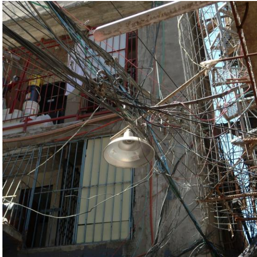
Figure 92. Informal and semi-formal electric connections in Villa 31.
