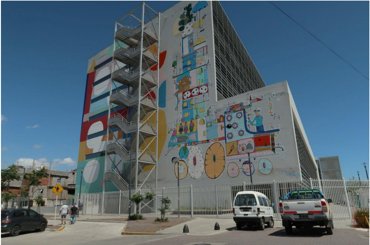
Figure 81. The new headquarters of the Ministry of Education of CABA in Villa 31
