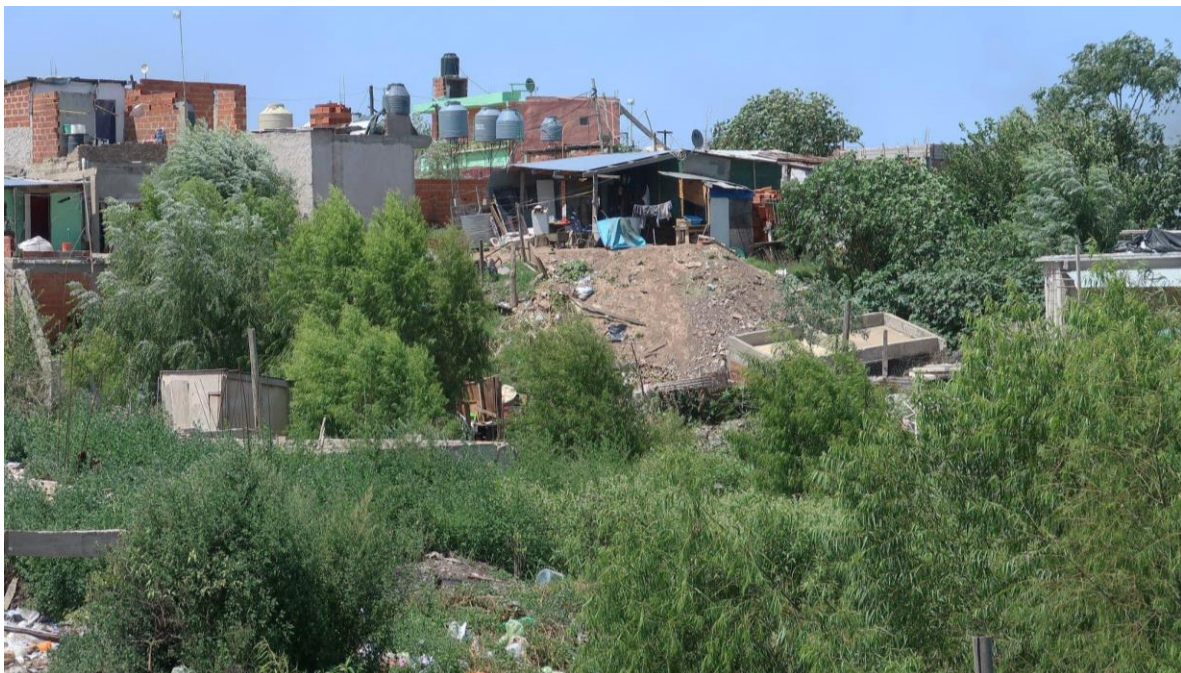
Figure 108. A house built with brick and reinforced concrete visible in the middle-right between the greenery has collapsed due to unstable ground.
