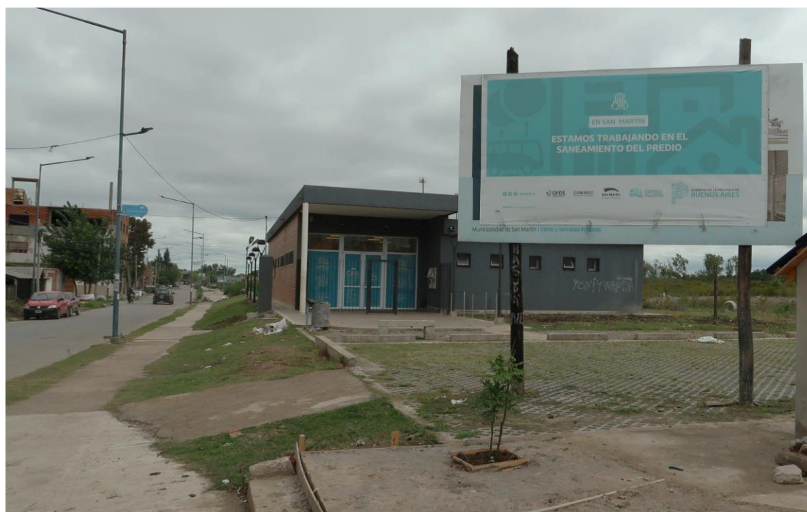
Figure 114. The Neighbourhood Service Centre (CAB) and a promotional board built by OPISU in Costa Esperanza
