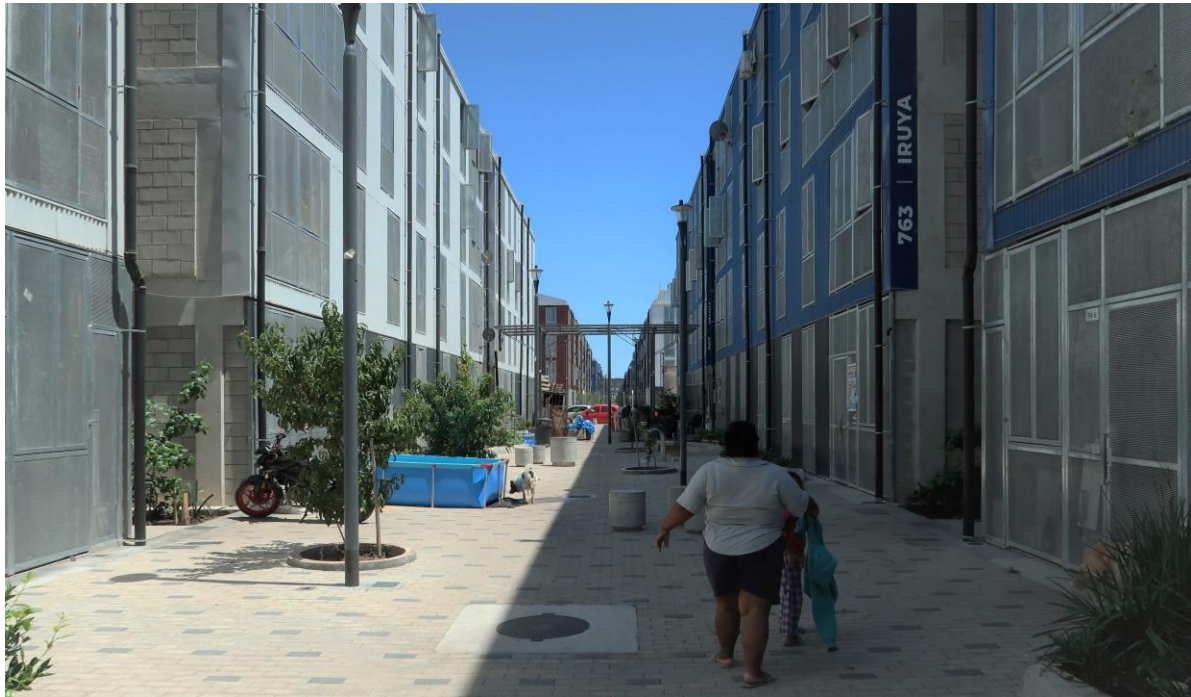
Figure 90. New housing in the YPF sector.
