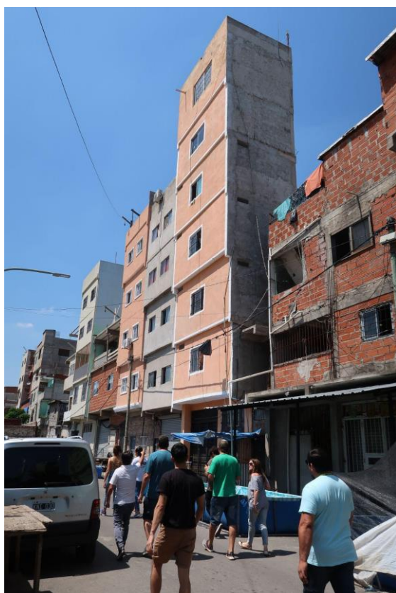
Figure 26. A 7-storey building in Villa 1-11-14.
