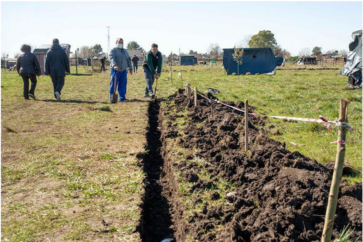
Figure 135. Neighbours collaborated to dig dikes and drains to mitigate flooding. Photo: Sebastián Linero (Enfoque Rojo)
