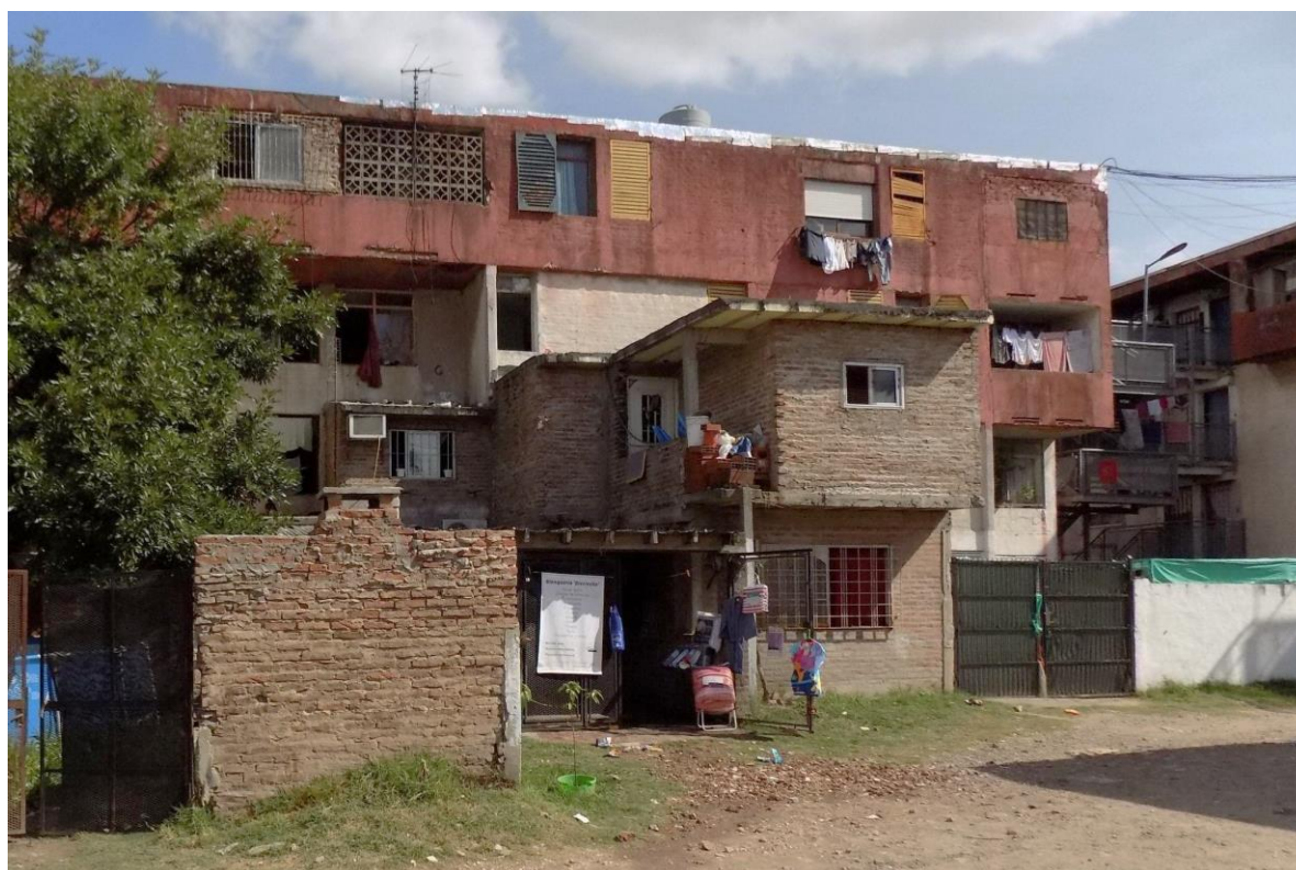
Figure 22. In the Carlos Gardel neighbourhood, new houses and housing extensions (front) were built in open spaces between the original buildings (back). This is an example of informalisation of a modernist housing project, which has gradually turned into a shantytown.
