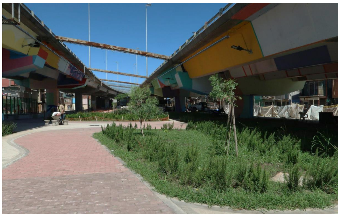
Figure 73. The first completed section of the park under the Illia highway.
