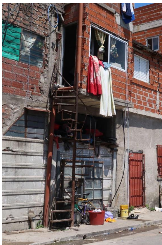
Figure 27. Spiral metal stairs in Villa 1-11-14.
