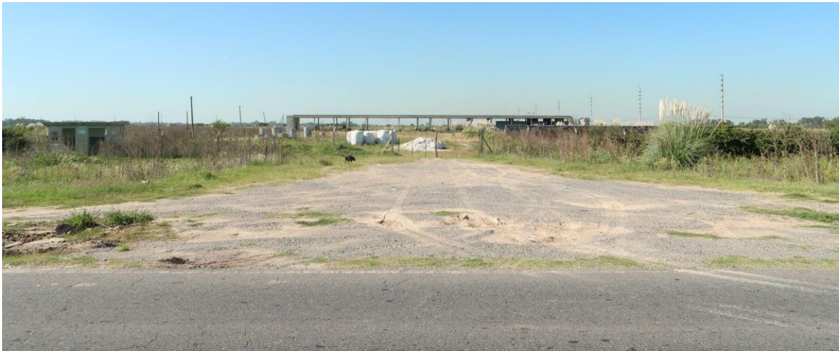
Figure 140. Entrance to the abandoned construction site of the San Cirano gated community project in 2022.
