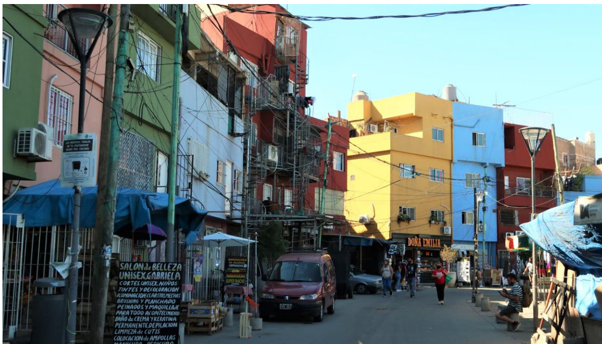
Figure 79. Facades of houses along this square have been improved and painted.
