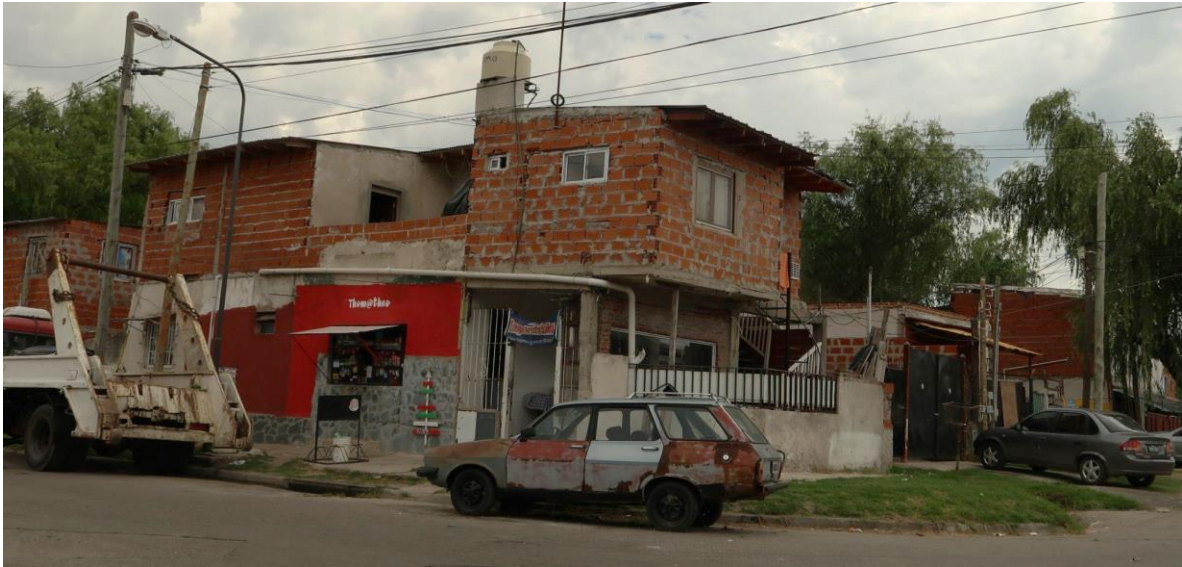
Figure 47. Incremental expansion of a house with a commercial unit on the ground floor in an informal settlement Juan Pablo II in Tigre partido.
