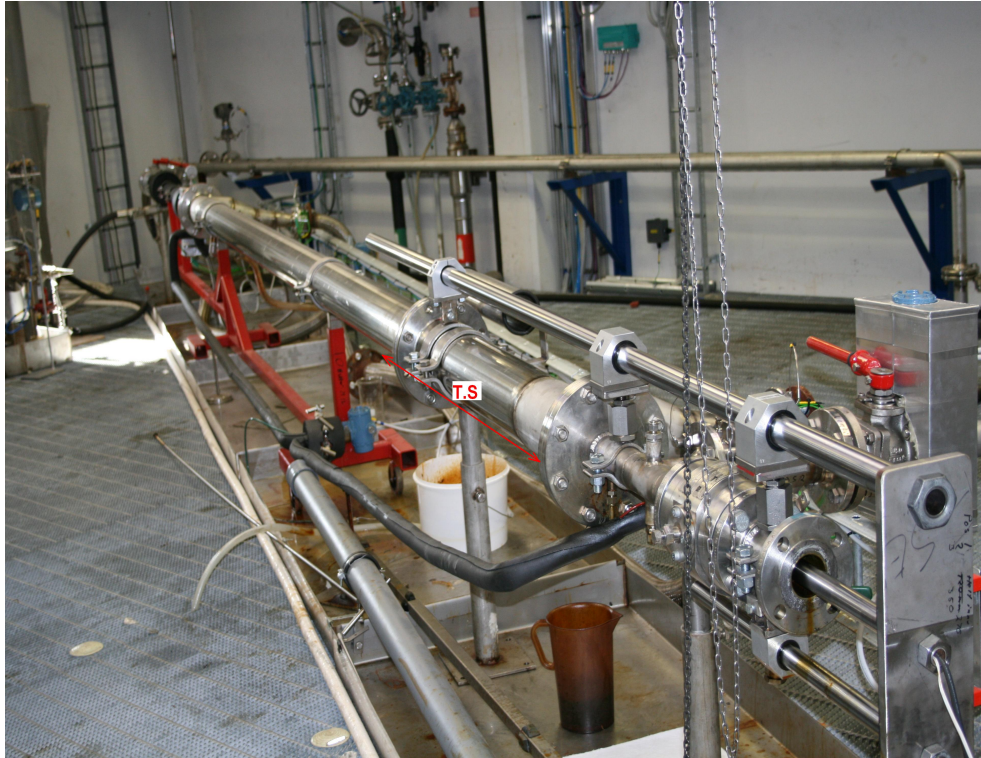
Figure 4.2: Picture of the facility
