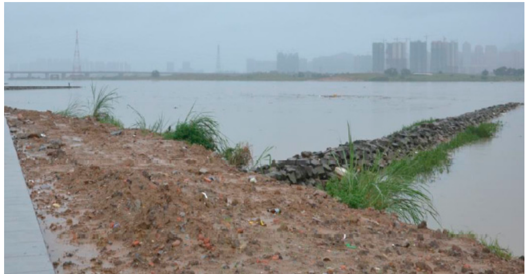
Figure A2. Spur dike in NG section.
