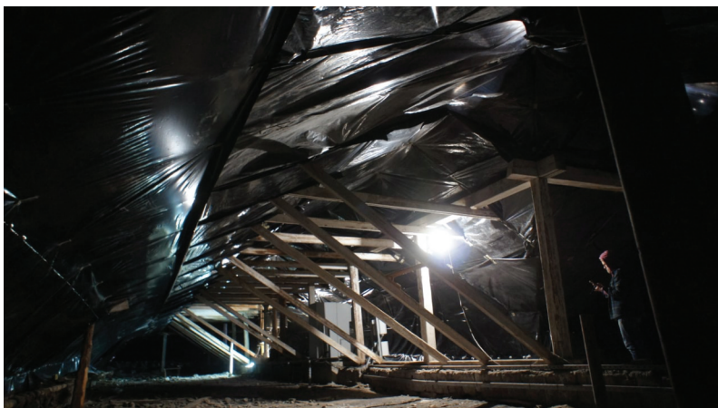
Figure 2. Repair works of Fabrika's roof. Photo by Yuren, December 2022.
