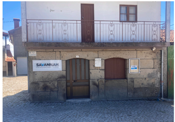
Fig. 9. Savannah’s Covas Information Point. “Savannah: Enabling Europe’s Energy Transition.” Source: Authors, 2022.
