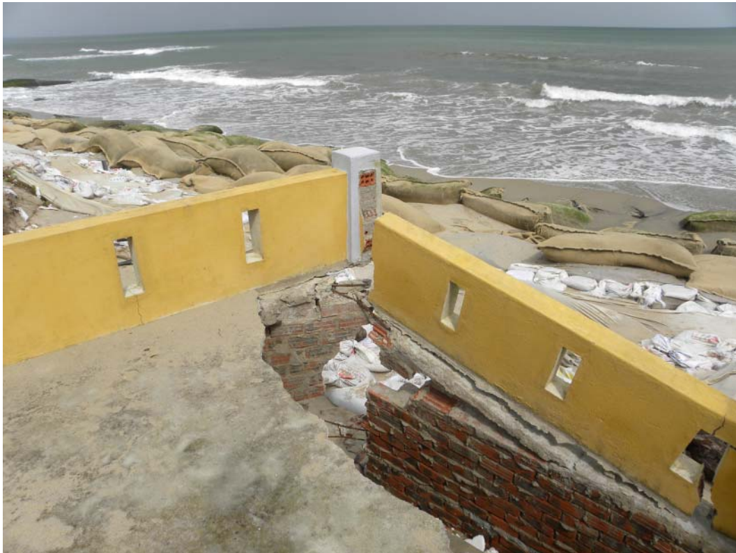
Figure 3. Erosion at Cửa Đại: sandbags on the beach and a collapsing whale temple. Photograph by Aike P. Rots, 2019.
