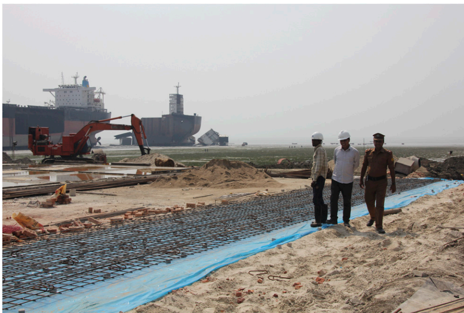
Figure 2. Image of PHP constructing impermeable floors. Sibilia, March 2016.
