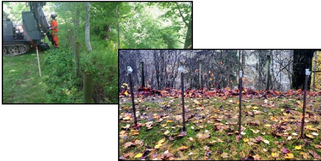
Figure 4-11. Left: A geotechnical drilling rig was used for the installation of the slope instruments (Heyerdahl et al., 2018). Right: Installed piezometers at 6m, 9m, 15m, and 23 m (photo during visit to the study area 3.11.22)
