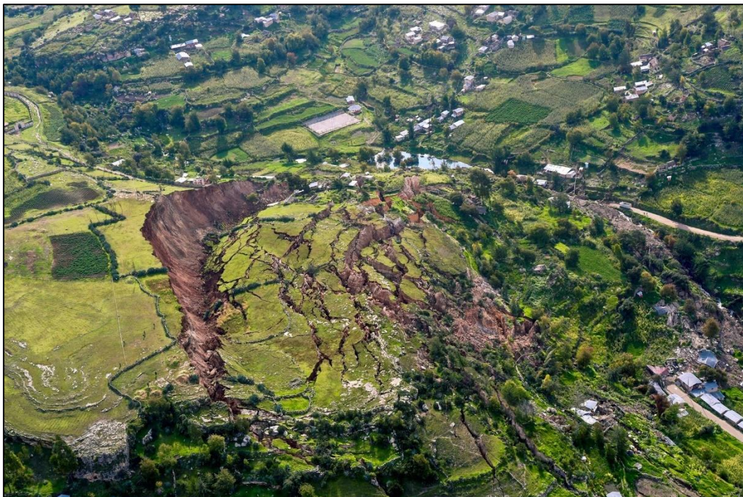
Figure A-7. A non-circular rotational failure that occurred in Cusco, Peru in March 2018. Most likely triggered due to high porewater pressures (Prince, 2019).
