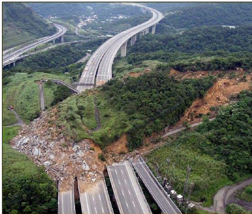
Figure A-5. A massive translational failure occurred in Taiwan in April 2010 (NBC News, 2010).
