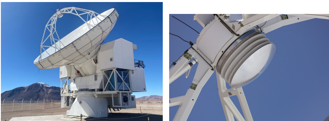
(a) Telescope structure. Credit: C. Cicone (2023) (b) Subreflector. Credit: P. Gallardo (2023)
