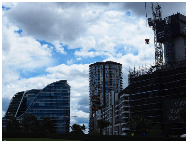
Figure 3: Construction and new apartments next to Green Square station. Source: Private photo
