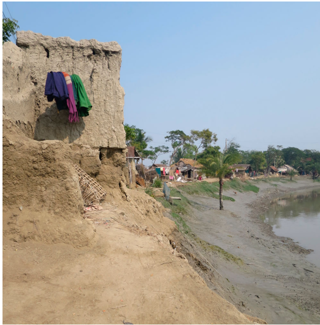
Figure 3. Riverbank erosion in Satkhira district January 2015. Photo by Author.
