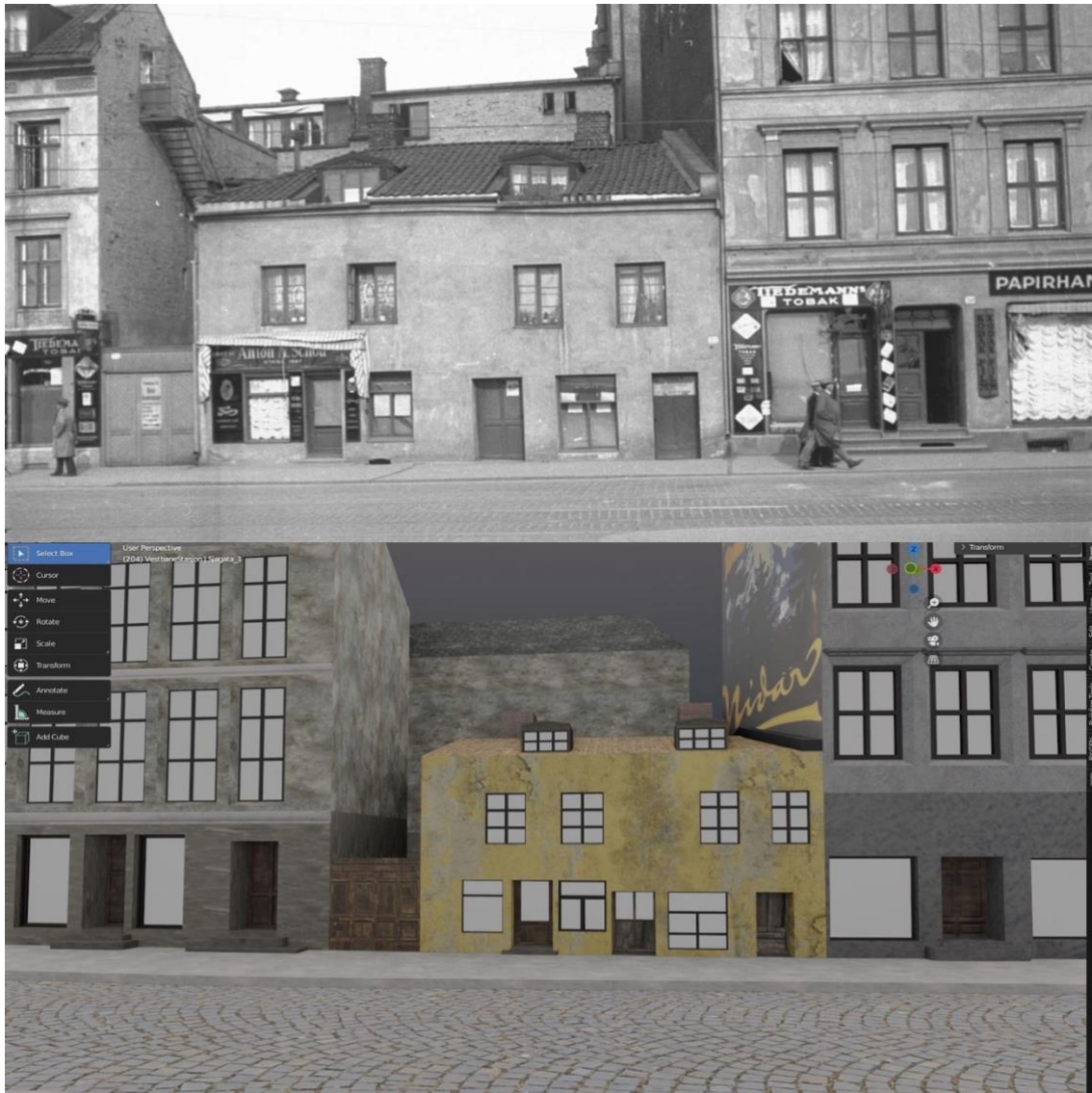
Figure 9: The yellow house. Sjøgata 22.
