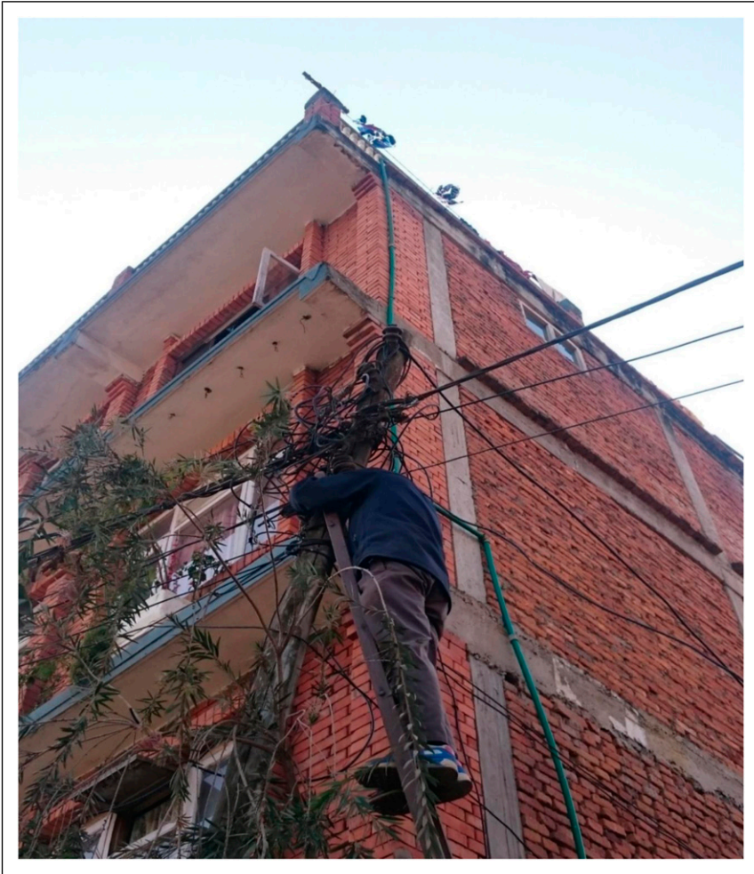
Figure 1. Connecting the cable to the main utility pole on the road.
